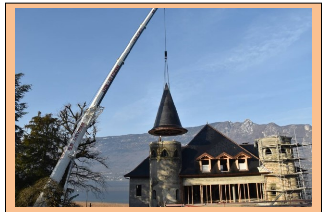
6 th stage: Roofing and then installation of the 2 conical frames with the help of a crane.
