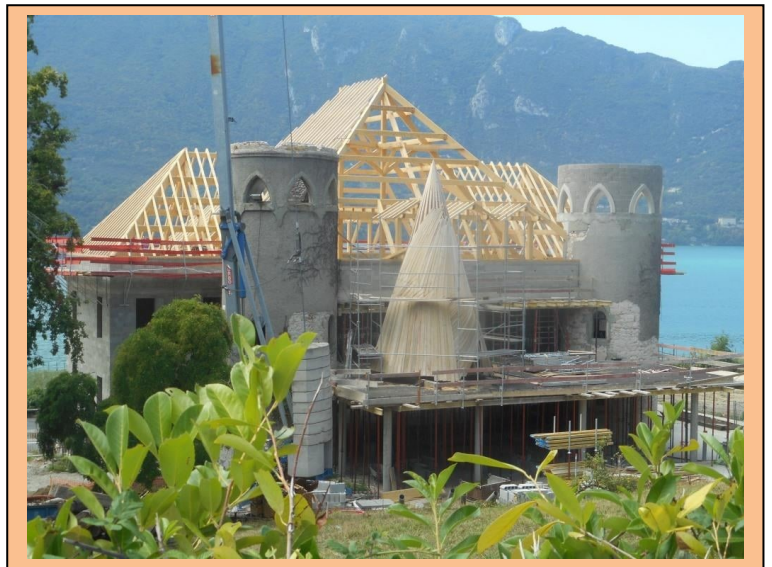
6 th stage: Roofing and then installation of the 2 conical frames with the help of a crane.
