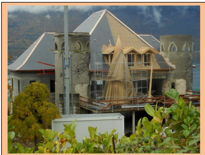
6 th stage: Roofing and then installation of the 2 conical frames with the help of a crane.
