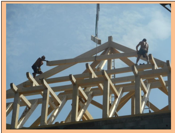
6 th stage: Roofing and then installation of the 2 conical frames with the help of a crane.
